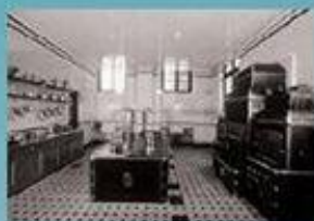
Le fourneau central de la cuisine de l'Hôtel Camondo. © J.-C. Dوتر, 2004 Camondo Mansion, main stove of the kitchen.
